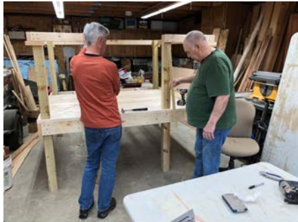
Bill Kelleher (left) and master carpenter John Currens review the progress of the Mount Baldhead observation tower that will be used in the upcoming exhibit.
